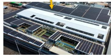
New Water Plant and FG
