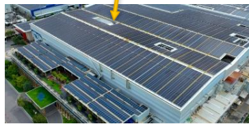
Head Office and Rooftop
